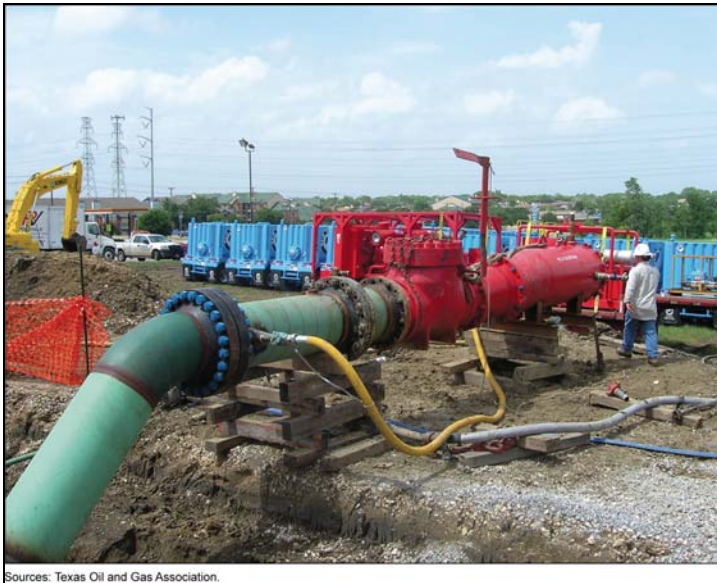
Figure 1: Hydrostatic Testing Equipment Used to Test Pipeline Integrity
